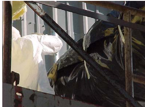
Temporarily secure film with common tape.
