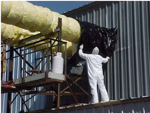
Wrap insulation with film.
