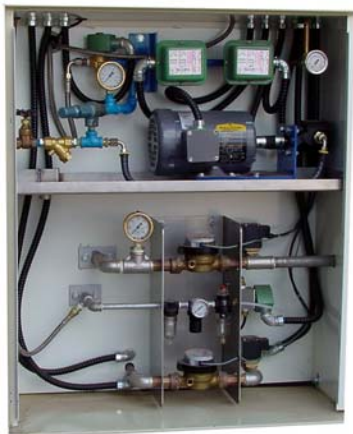
Fuel valve train and water metering
