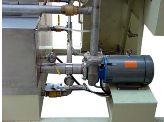
7-1/2 HP cast stainless pump delivers performance
