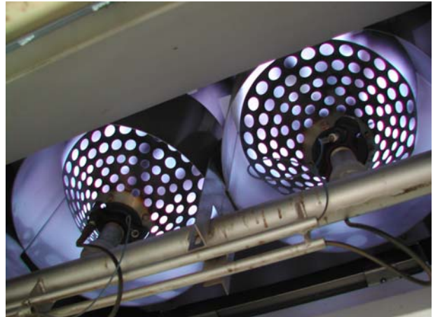
Dual 4-million Btu/hr gas burner heads provide 8-million Btu/hr of high air volume heating.
